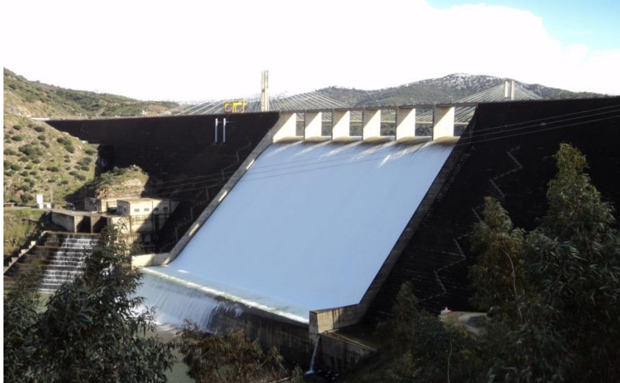
Figure II.5: Digue de Barrage Béni Haroun.
